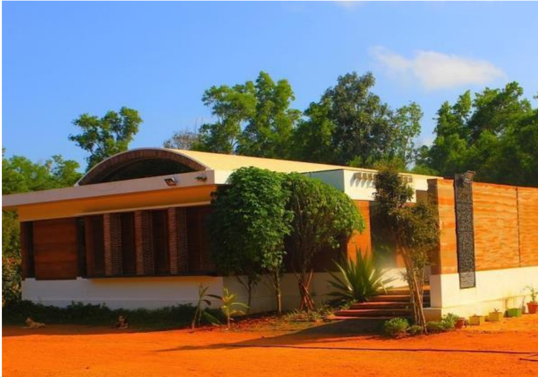
A private Guest house designed and built without NOC by Buildaur (Dharmesh, Dhruv and their team) in the Master Plan (GB)
